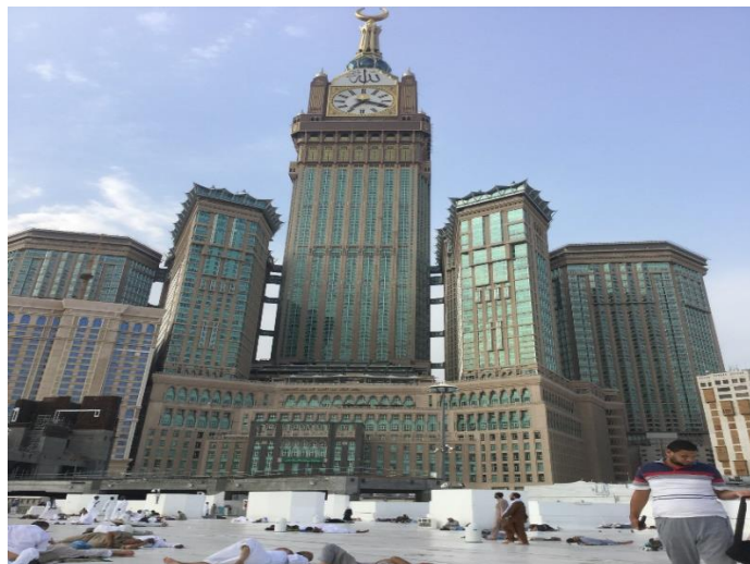
Fig. 1. Royal Clock Tower building from roof top of Masjid al-Haram Mecca, note the surrounding buildings with connecting corridors.
